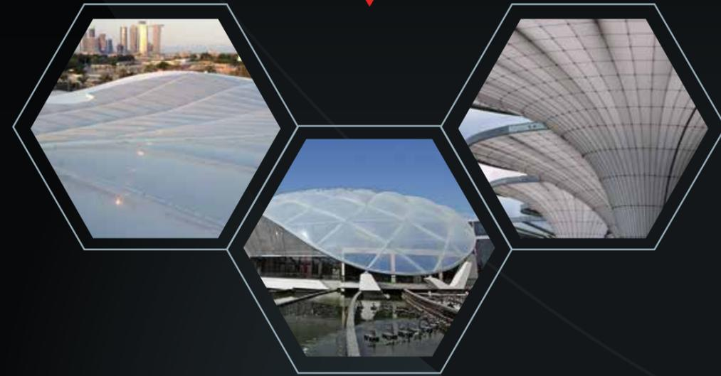
Ethylene TetraFluoroEthylene (ETFE) is a fluorine-based plastic which is lightweight, transparent, recyclable and strong. It weighs only 1% of an equally-sized glass panel and makes comparative energy savings of around 30% as it lets in more light and is a better insulator of heat. ETFE is also dirt and wear resistant and can be kept clean by rainfall.
